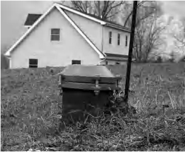
Figure 2.3. A sanitary well cap installed on a well casing.
