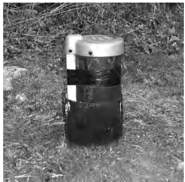
Figure 2.2. A standard well cap similar to those found on most Pennsylvania wells.
