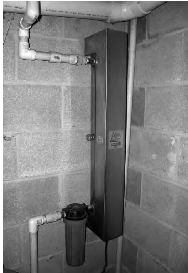
Figure 5.3. A typical UV light installation with a small canister sediment filter ahead of the UV light unit.
